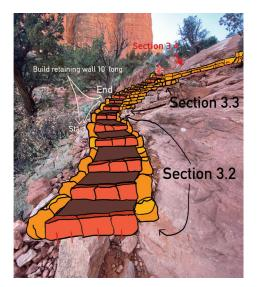
Local sandstone and limestone (weighing around 160 lbs per square foot) was quarried onsite from local gullies, then hauled uphill using various methods, depending on the size and destination of the rocks. Several 300-pound boulders were hoisted 400 linear feet and 80 vertical feet uphill via a special grip hoist and gas winch.
